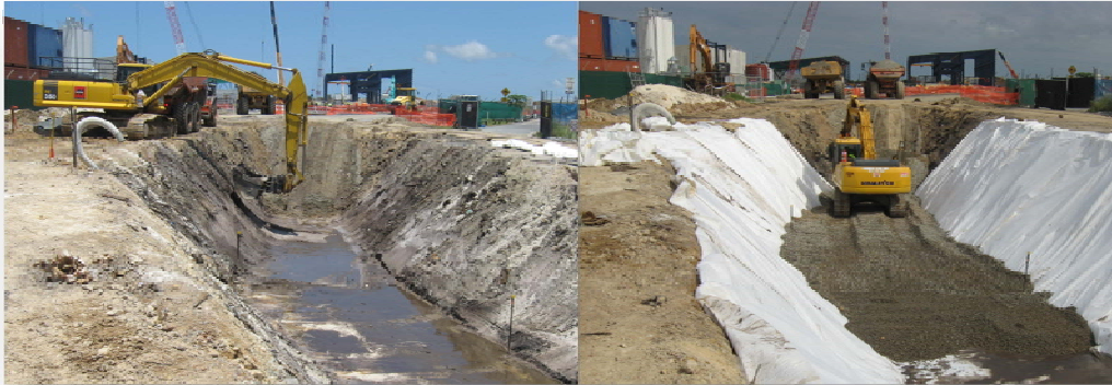
Installation of specific design aspects to control landfill gas and leachate
